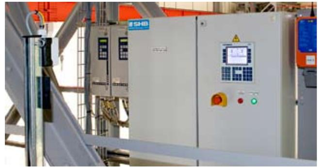
*The Emotron electronic flange control ensures fully synchronized travelling. The auto tune function of the crane control system means no PC is needed. Parameters and settings are clearly displayed.*
