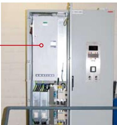
The choice of drive solution was a fully digital DC drive from Emotron, developed especially for modernizing high-speed lifts while retaining the original DC motor.
