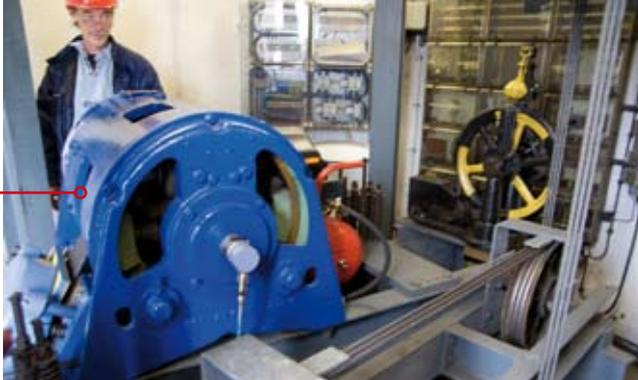
The project was complicated by the fact that the motor is located in the machinery room at the top of the tower and the DC converter is at the foot of the lift shaft. This requires a motor and encoder cable measuring 220 metres.
