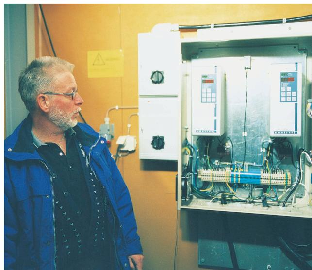
*Electrical installation is extremely easy and cheap with the built-in safety functions. A small electrical cabinet is all that's needed for a complete system with monitoring and remote alarm via mobitex.*
