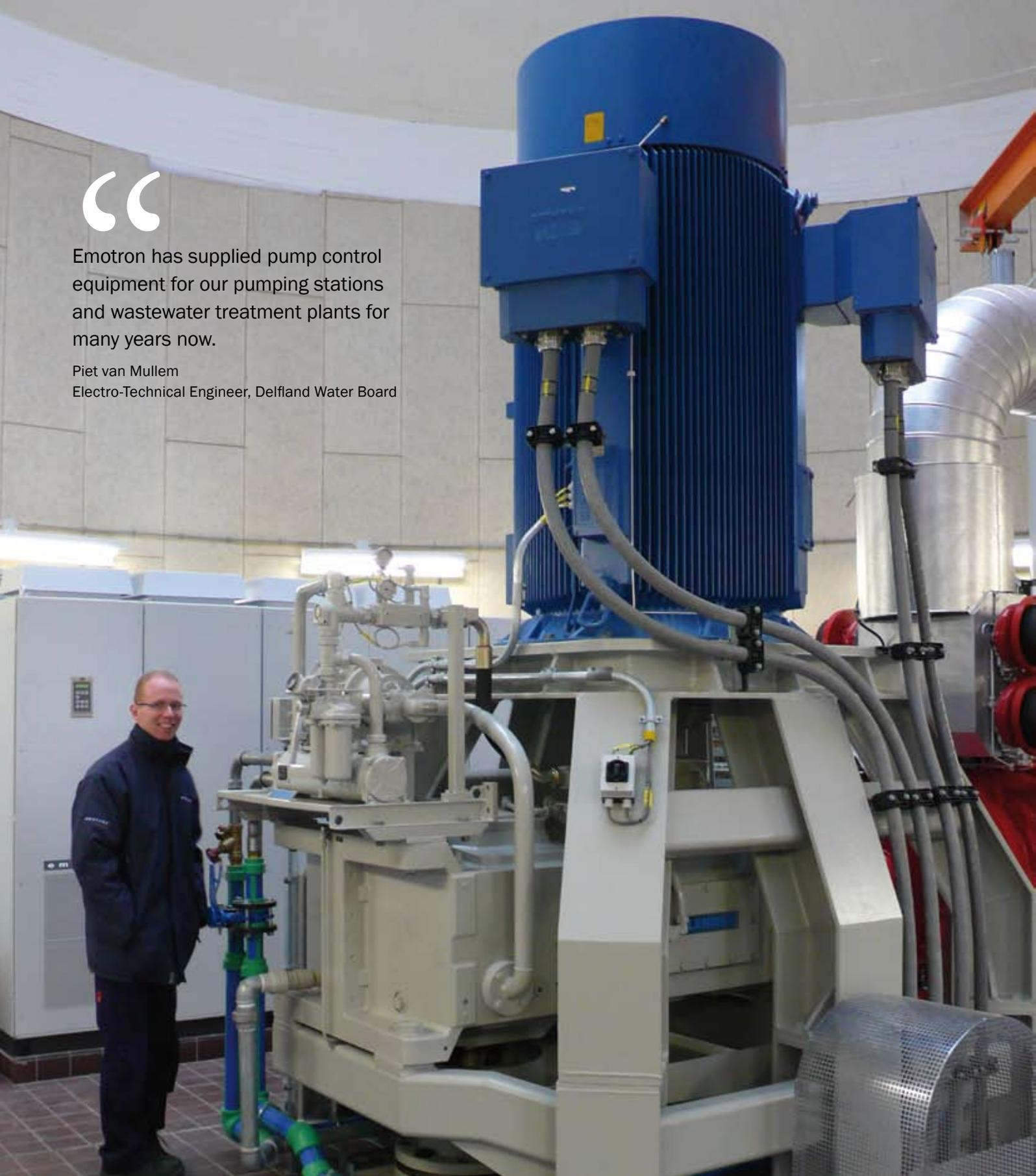
*Emotron and Bosman Watermanagement upgraded the pumping capacity of Parksluizen pumping station from 10 m<sup>3</sup>/s to 20 m<sup>3</sup>/s. The IP54 classified Emotron FDU variable speed drive is installed next to the Bosman Beveron 210 pump. Service technician John Derks from Emotron worked on the installation.*
