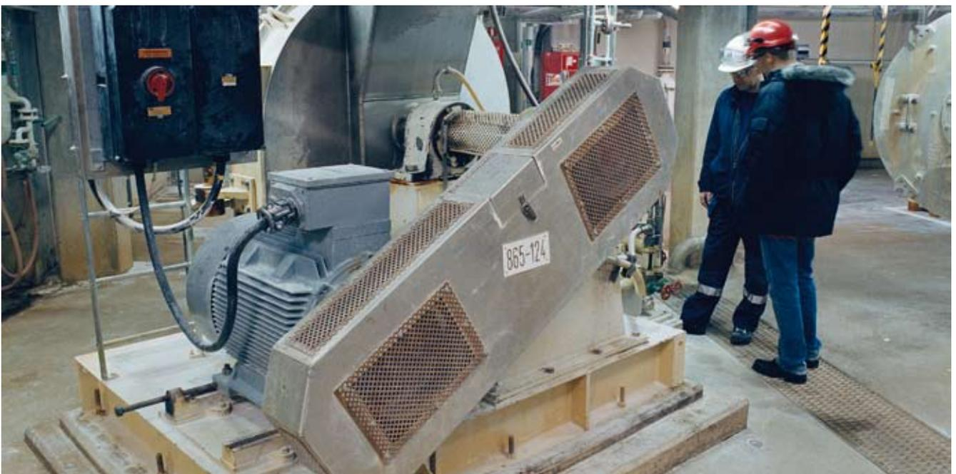
*It is important that the grains of PVC powder are the right size. Any powder which needs more milling passes through a mill controlled by an Emotron variable speed drive. "We usually use the comparison with potato flour to describe how fine the powder should be," says Martin Ljungqvist.*
