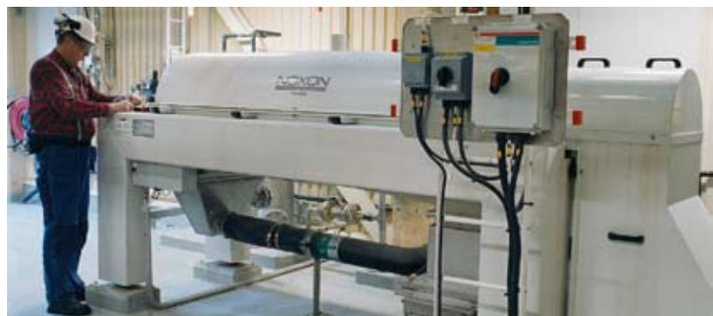
*Operator Gary Karvinen working on a sludge centrifuge in the waste water purification plant. The centrifuge is controlled by an Emotron variable speed drive, as are the blowers which oxygenate the waste water.*
