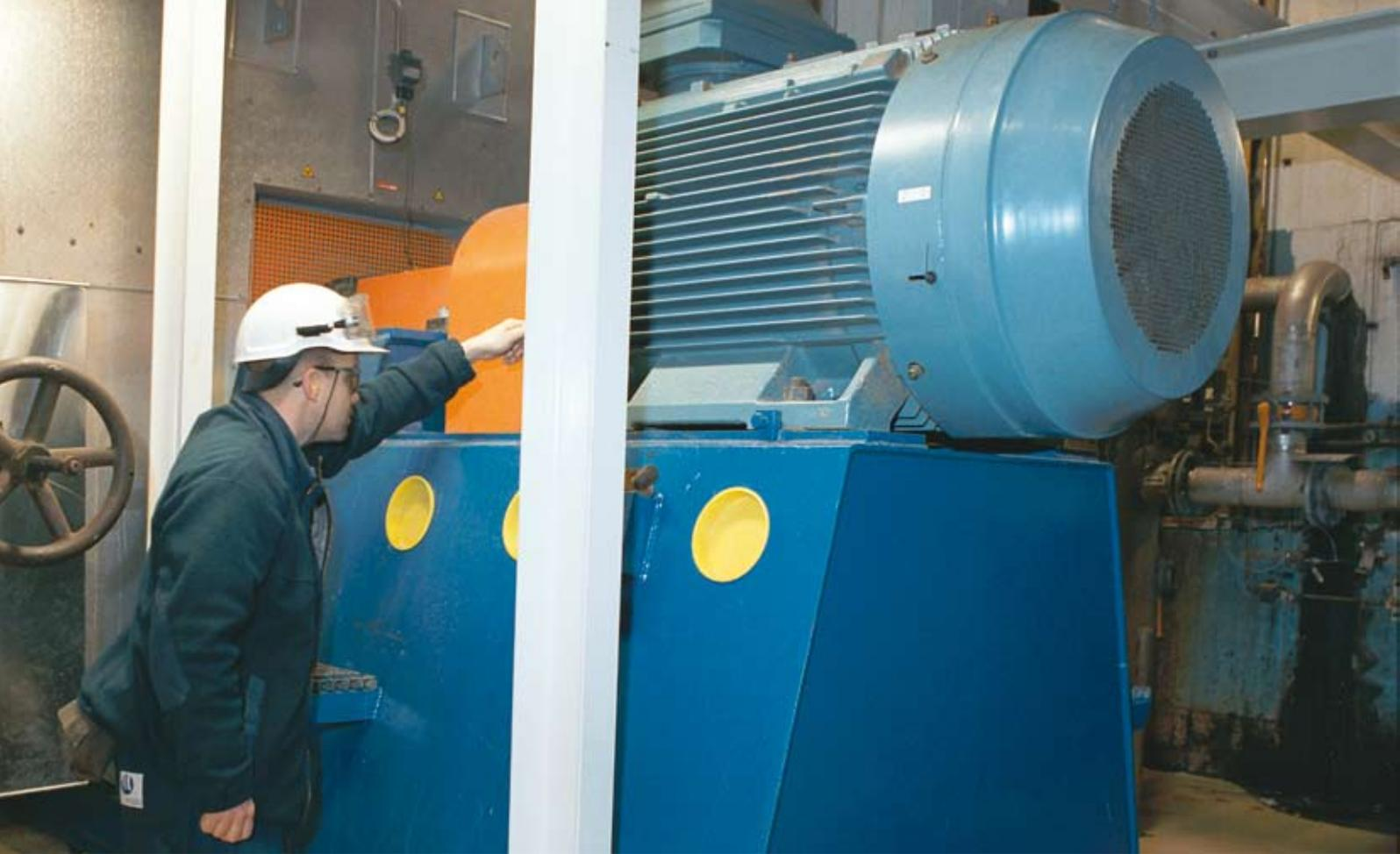
*Martin Ljungqvist, the supervisor of the electrical department at Hydro Polymers, checking one of the flue gas fans in the boiler room which is controlled by Emotron variable speed drives.*
