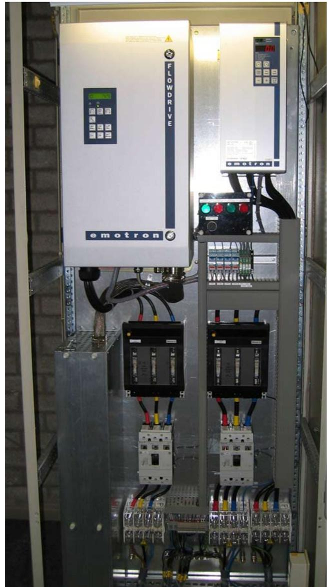
*In the new set-up, however, the pumps are started up using an Emotron FDU frequency inverter and an Emotron MSF softstarter respectively and are controlled by a pump control fully integrated in the frequency inverter.*
