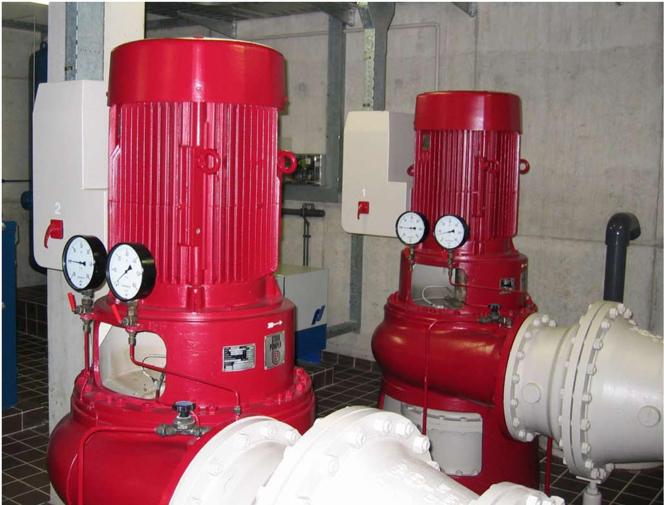
**The flush pump system at the Lith drinking water production plant, a division of Brabant Water, recently underwent an overhaul. This system comprises two 55 kW centrifugal pumps driven by electric motors. They produce a combined output of 0 - 2000 m<sup>3</sup>/hour.**
