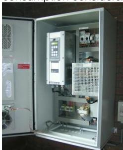
*Emotron variable frequency drives (AC drives) in combination with an all-pole filter.*
