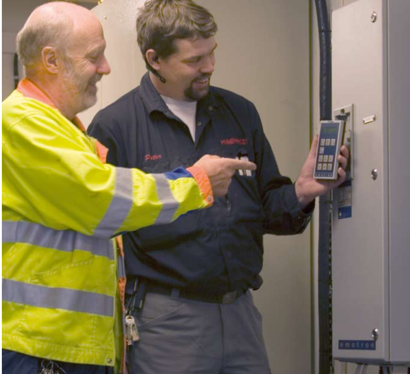
Pumphuset chose Emotron's new FDU 2.0 variable speed drives for control systems at Sollentuna Energi. "Installation is simpler and cheaper thanks to the smaller size and higher enclosure class. The removable control panel means it's easy to transfer settings," say Peter Johannisson (r) and Franc Rostedt (l).
