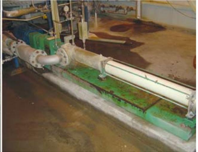
Emotron M20 monitors protect progressive cavity pumps (on the left) and magnetic drive centrifugal pumps used in the ISP Calvert City chemical plant.
