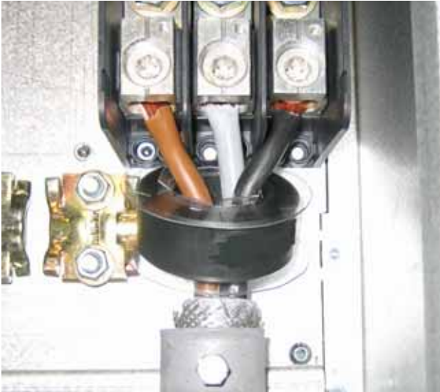
Fig. 55 Ferrite core mounted on the motor cables
